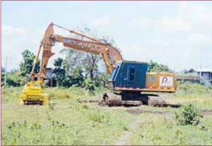
PRO MAC BDM 48 attached to a CASE 9040 B excavator
